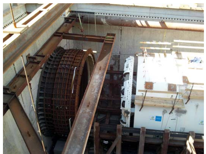
Fig. 3: TBM during set-up and assembly in the launch shaft
