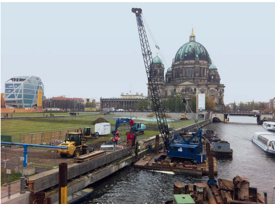
Fig. 4: Pulling up sheet piles
