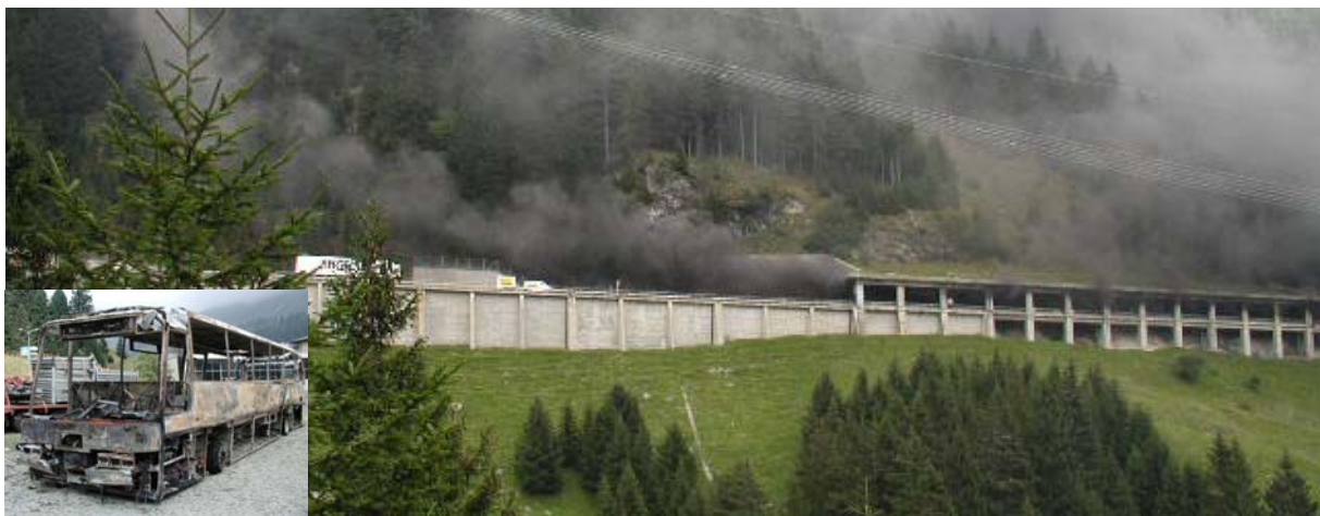
Figure 7: Smoke propagation during a bus full fire (2002). View of the upper gallery portal and image of the bus after the fire in the inlay at the left lower corner.
